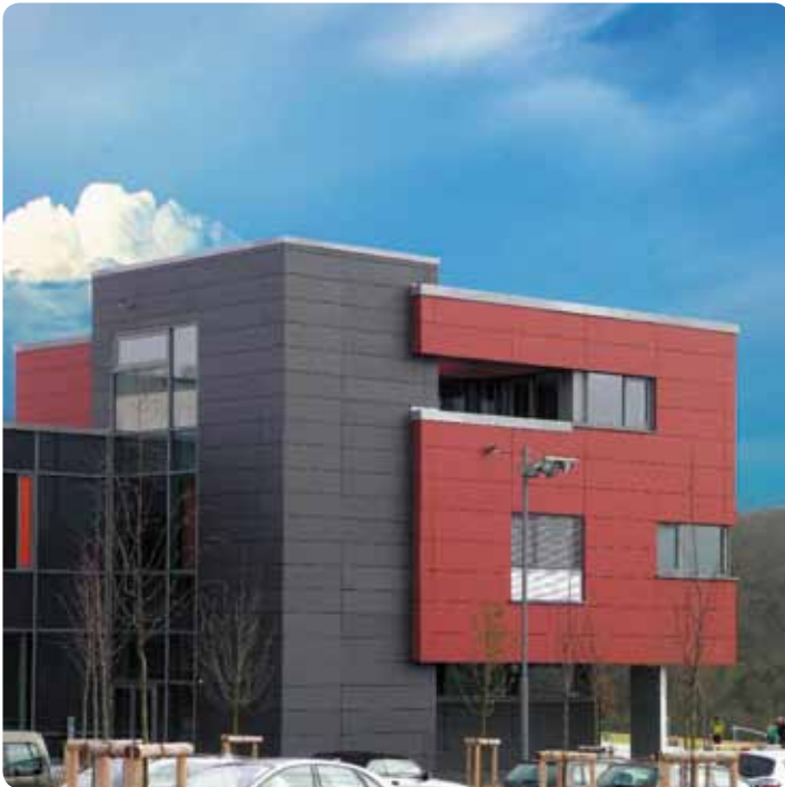
OFFICE BUILDING, REDANGE, LUXEMBURG (PHOTO: ETERNIT BELGIUM)
