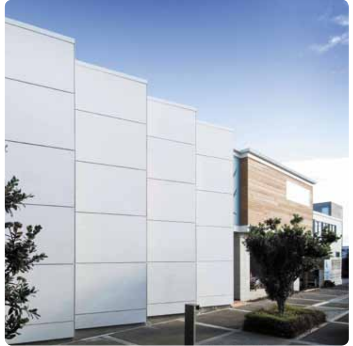
RESIDENTIAL BUILDING, NEW ZEALAND (PHOTO EURO PANELS)
