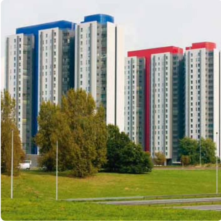
SILVERTOP, RESIDENTIAL BUILDING, ANTWERPEN, BELGIUM (PHOTO ETERNIT BELGIUM)
