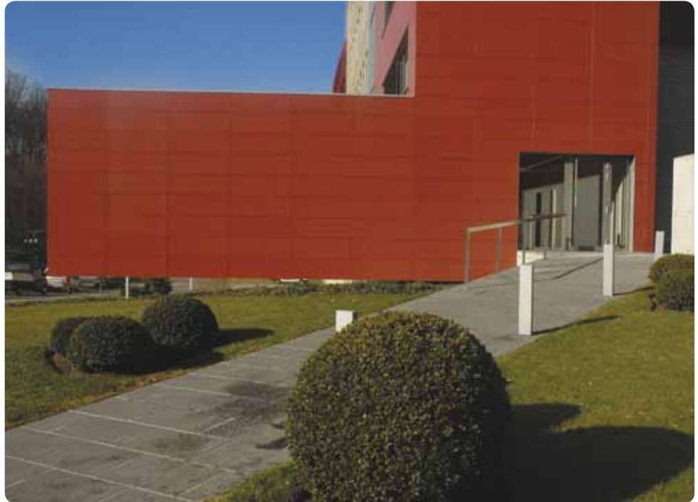
PROJECT LEUDELANGE, LUXEMBURG (PHOTO ETERNIT BELGIUM)
