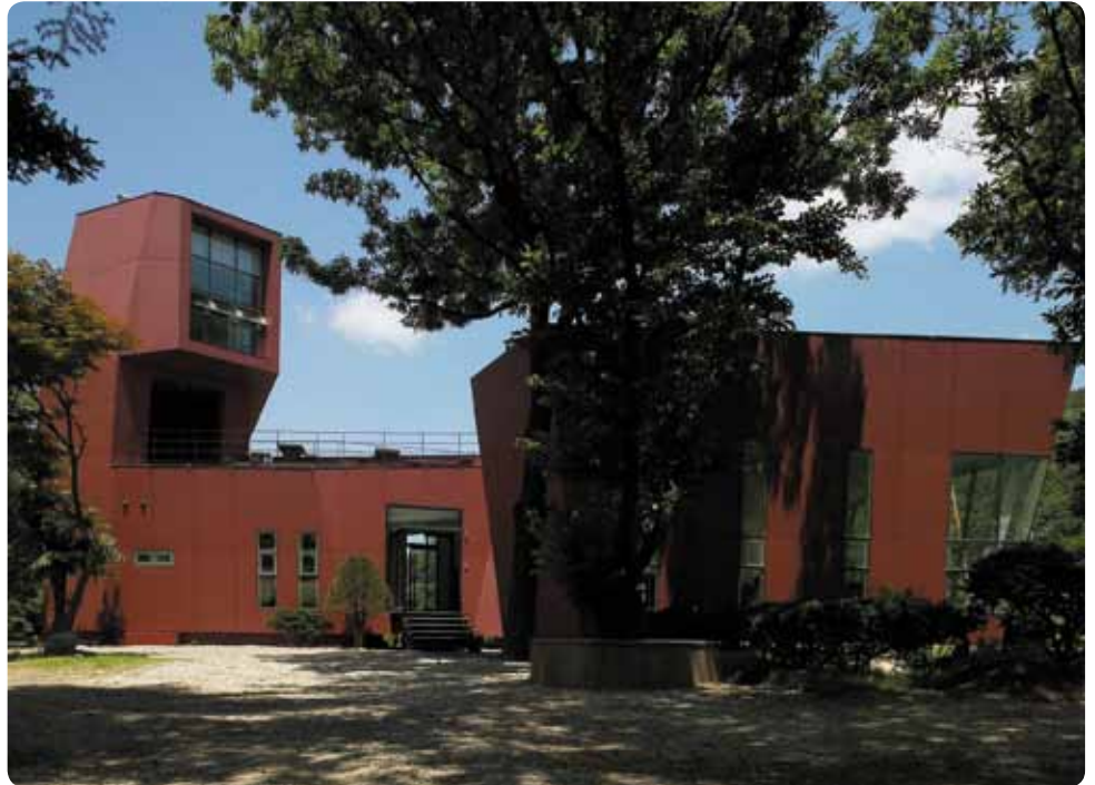
OLYMPIC FARM HOUSE, SOUTH KOREA (PHOTO: CHAI SU-OK)
