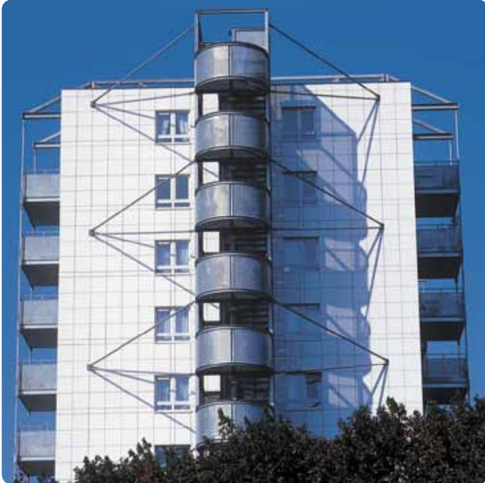
ZONNEVELD, THE NETHERLANDS (PHOTO: ETERNIT BELGIUM)
